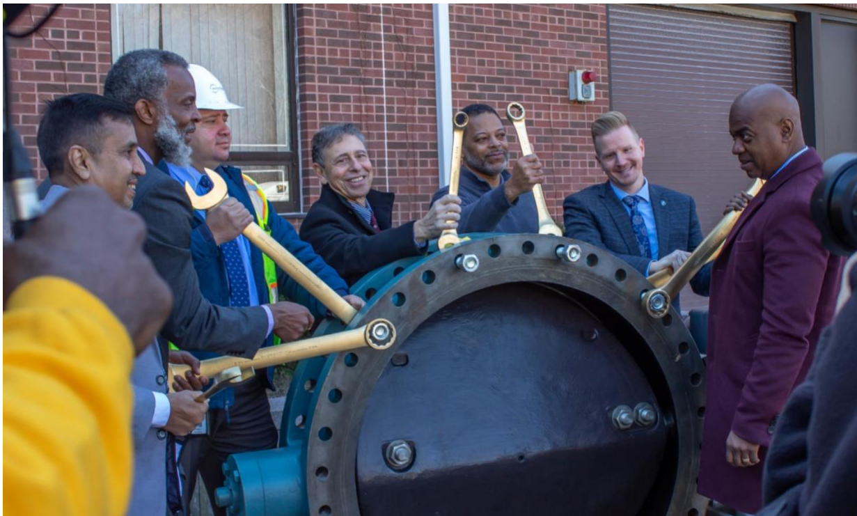
Newark Mayor Ras J. Baraka was joined by DEP Commissioner Shawn M. LaTourette, Licensed Operator of Treatment and Distribution, Jerry Notte and Newark Water & Sewer Utilities Director, Kareem Adeem to celebrate the launch of $23 million in new upgrades for a facility at the Pequannock Water Treatment Plant in West Milford, New Jersey.
