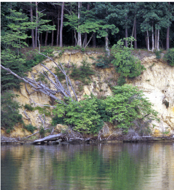
Coastal erosion causes shoreline collapse (photo by Chesapeake Bay Program).
