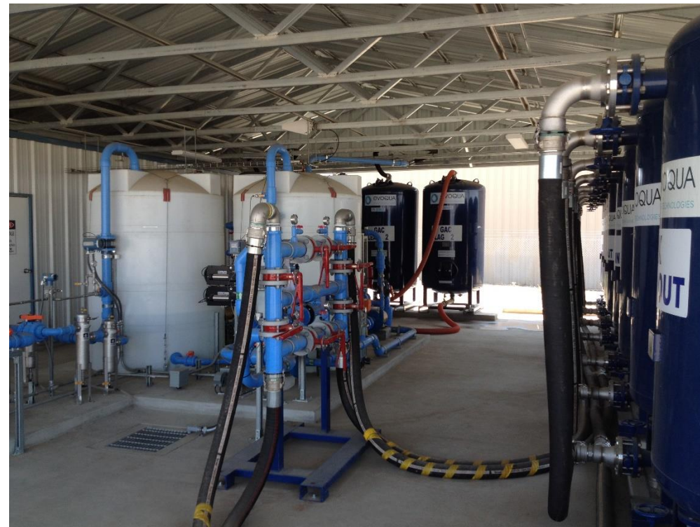
GAC/IX system treating 80 gallons per minute (for 123-trichloropropane in this case)
