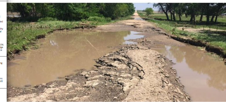
Road 5600 north of road P in the county on 05-30-19
