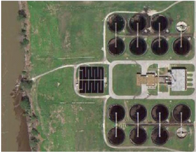
M.C. Stiles Plant
