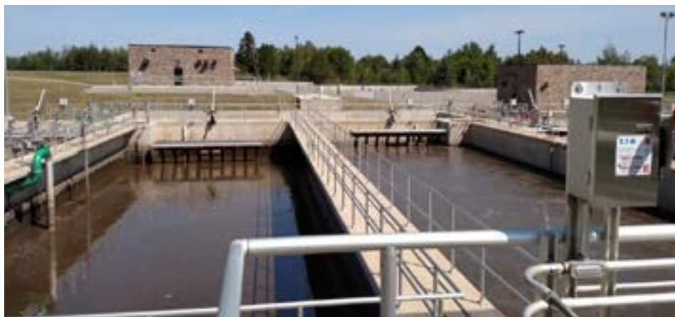
Sequencing Batch Reactors. Photo Credit: Central Iron Range Sanitary Sewer District
