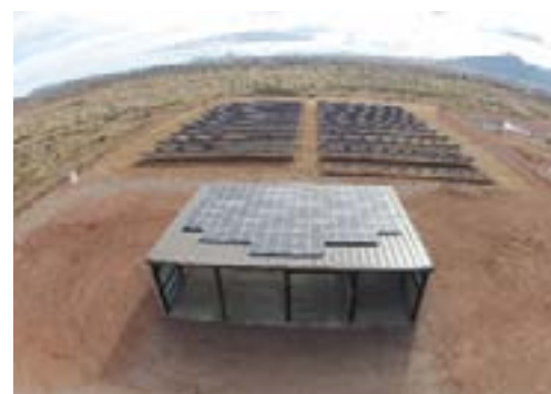
Views of the 400-kilowatt Solar Array at the San Jose Wastewater Treatment Plant. Photo Credit: WIFA of Arizona
