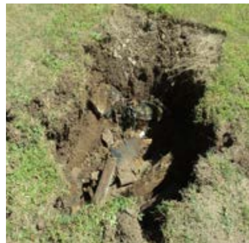
An Old, Collapsed Septic Tank. Photo Credit: Missouri DNR
