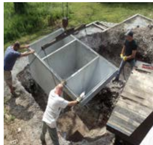
Setting a New Treatment Tank. Photo Credit: Missouri DNR
