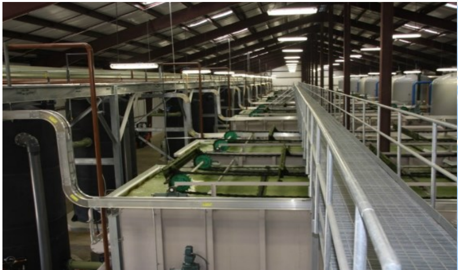
Algae Removal Process by Dissolved Air Flotation Units. Photo Credit: City of West Monroe
