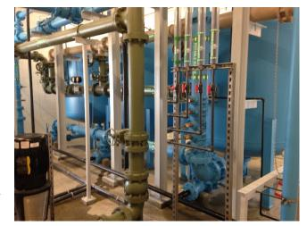
and installed by EPA staff. Tests demonstrated the system's ability to effectively remove ammonia and iron from the community's source water. A full-scale water treatment plant was completed in January 2014 based on the successful pilot system.
