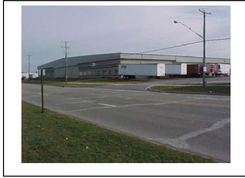
After: One of three 120,000 square foot warehouses.
