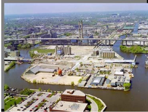
Before: The DPW yard contained underground storage tank and salt storage.
