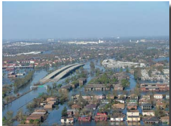
Flooded roadways in New Orleans East.
