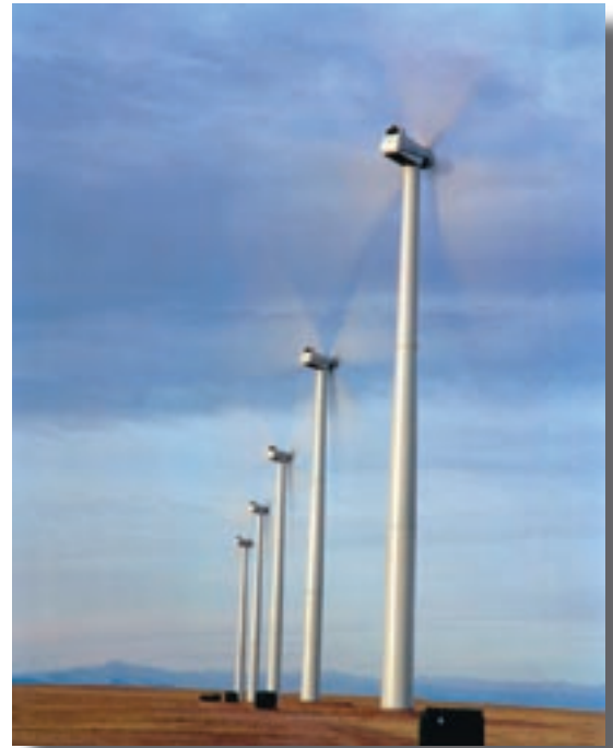
The Colorado SEP supports emission-free wind power. Pictured here is the Ponnequin Wind Farm in Colorado.
